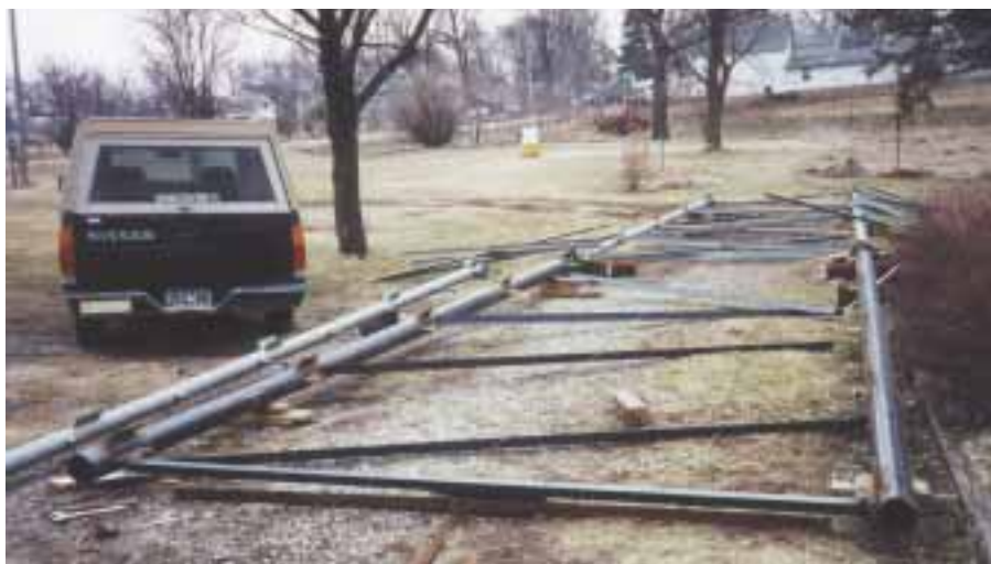
The homebuilt base section's geometry was extrapolated downwards from the Rohn's original bottom section. The structural design was the same.
