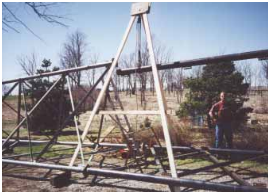
The 40 foot sections were assembled horizontally. Tripods, a winch, and block and tackle were used to position the 300 pound legs for welding.
