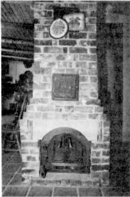
Above Left: Colin built this monster woodstove into the chimney's east end. Above Center: the wood cookstove is built into the chimney's westend. Above Right: with a large garden, the Sun Frost RF-12 stores many home-grown veggies.
