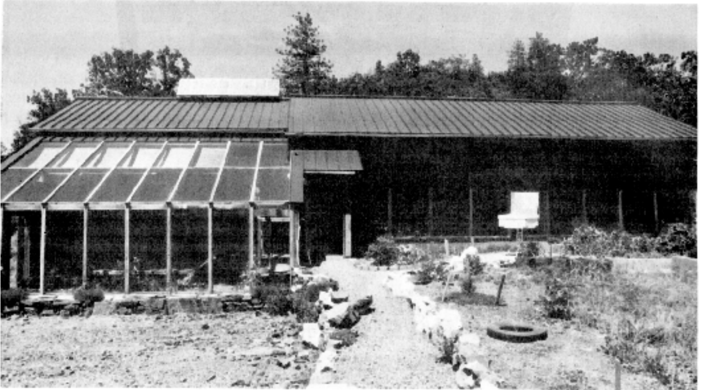
Above: a view of the south side of Colin and Christine's home. Large south facing windows and a greenhouse heat the home with sunshine. Photovoltaic modules on the roof provide the electric power. The solar oven in front of the house is baking bread. Photo by Richard Perez.
