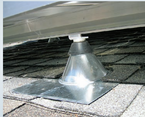
Oatey flashings provide a watertight seal for the mounting post.
