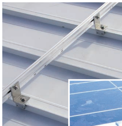
Top-down rail mounts are popular in both home- and business-scale installations.
