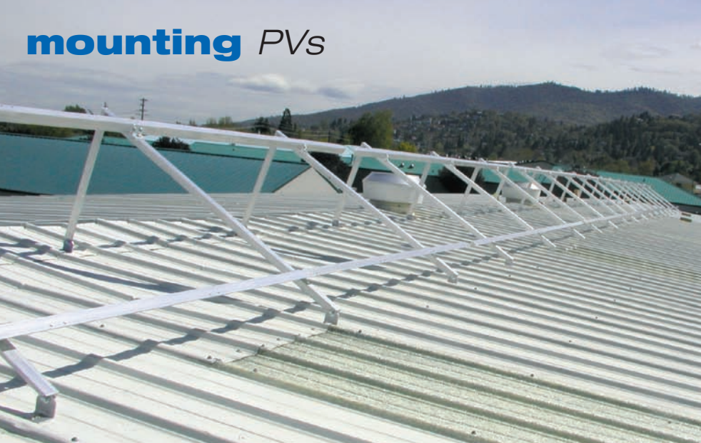
A DP&W rack sets an angle steeper than the roof pitch. Fixed-pitch and adjustable racks are available.
